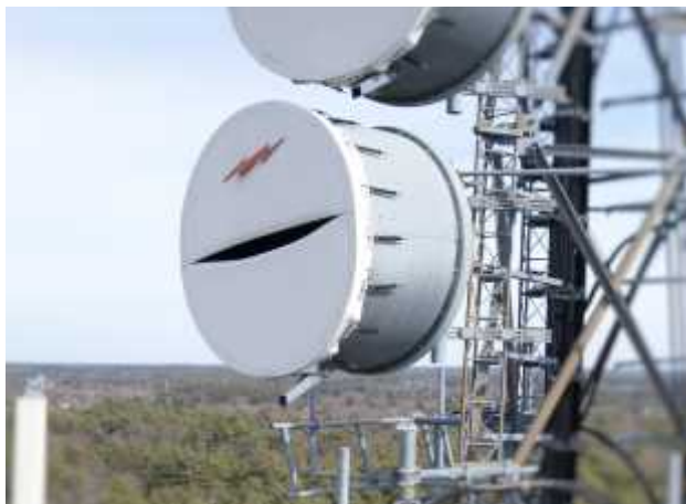
DAMAGE ASSESSMENT - CELLULAR TOWER
