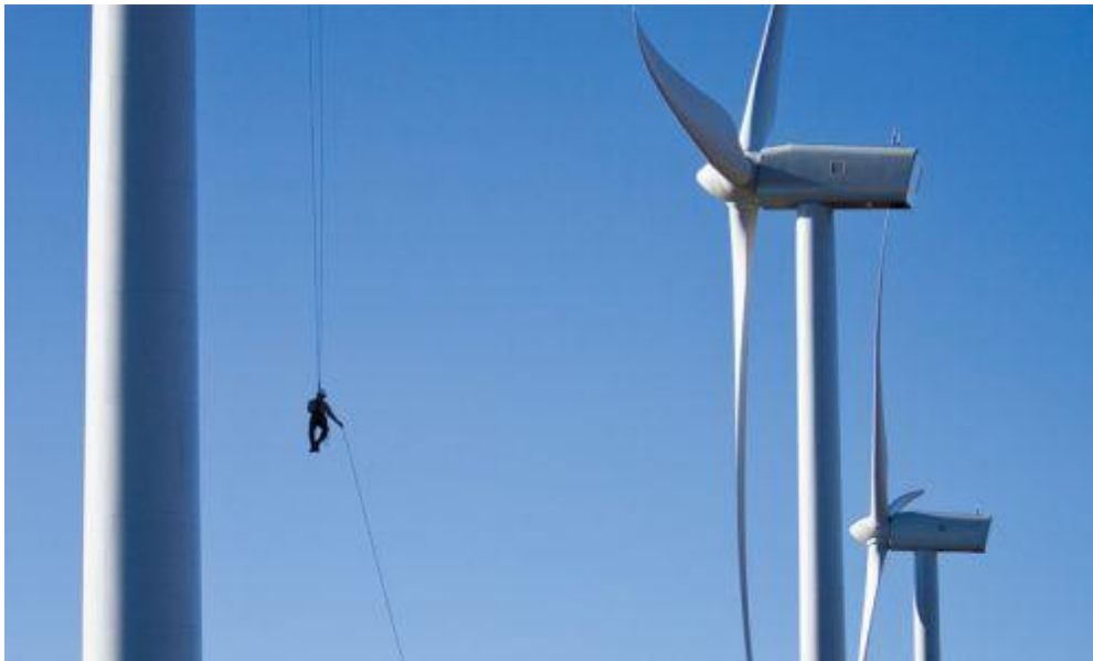
Figures 4 & 5: Photos of Current Rope Access Inspection Techniques
